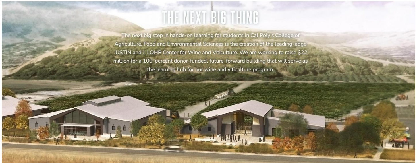
Center for Wine & Viticulture – Building 156 – the building is on the left
